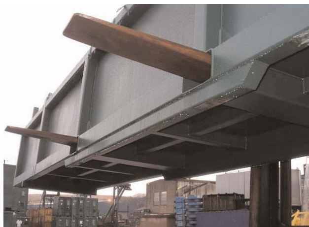
Typical Forklift Pockets.
