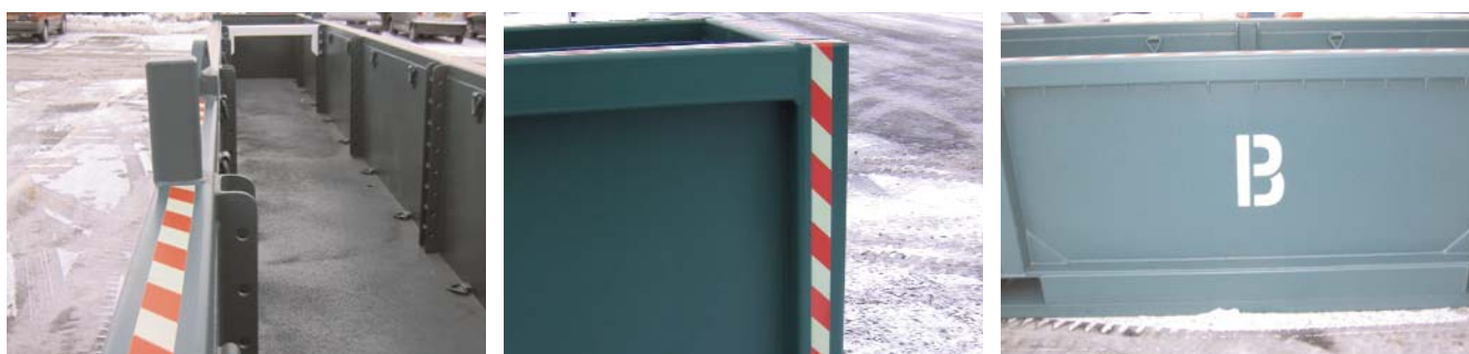
Examples of safety markings and stacking information identification.
