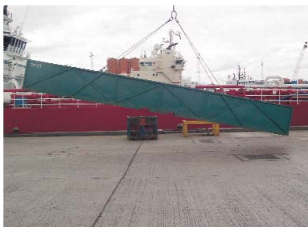
A lift showing an unacceptable unbalanced load.
